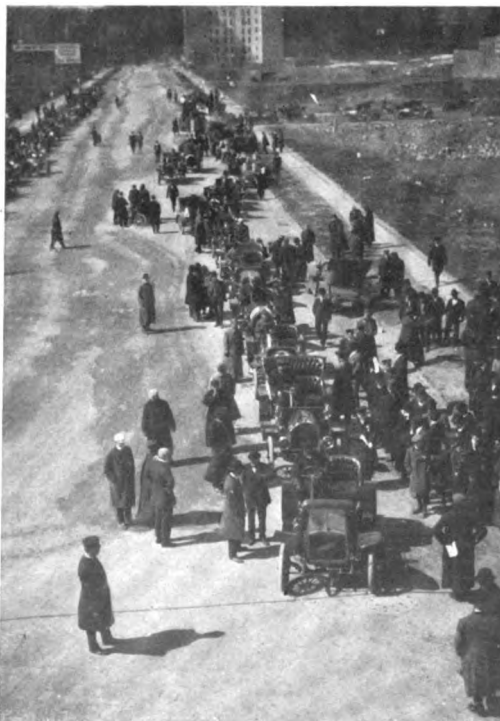
Starting at the Bottom of the Grade.
